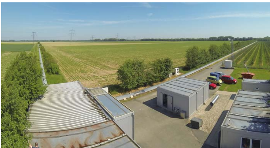
The GEO600 site in Ruthe 20km south of Hannover, Germany.
